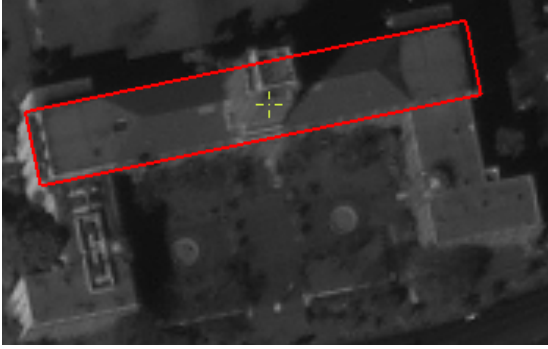
Figure 7. The building after the initial rectangle.
