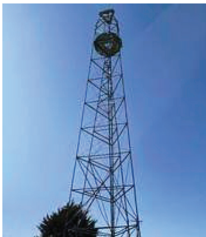
Figure 10. Bilby tower with internal tower (for instrument) isolated from external tower (for surveyor). NOAA Photo Library.
