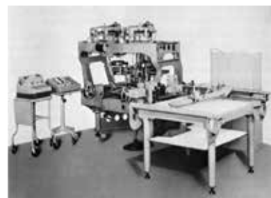
Figure 18. Wild A-7 stereo plotter with drafting table that I used to study photogrammetry at OSU. Here, only one stereo pair at a time underwent relative orientation. Although this had advantages, absolute orientation was harder to perform after bridging between multiple stereo pairs, one at a time. Source: Personal image.
