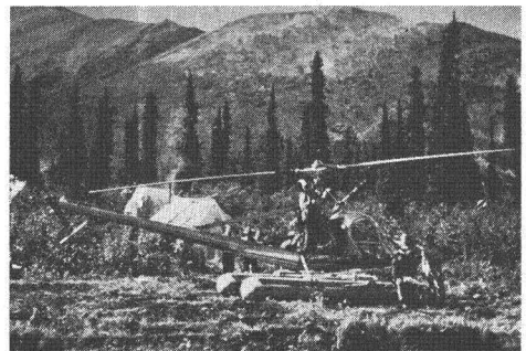
FIG. 2. The Base Camp & Landing Area at Elliott Lake, Yukon Territory.
