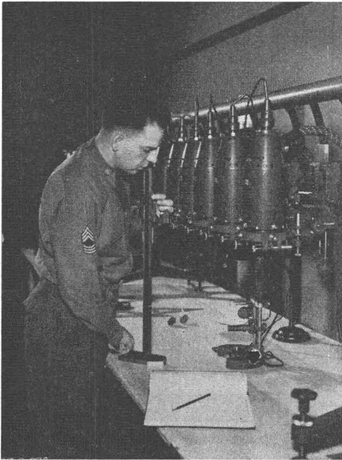
FIG. 8. Measuring Multiplex Projector Heights.
