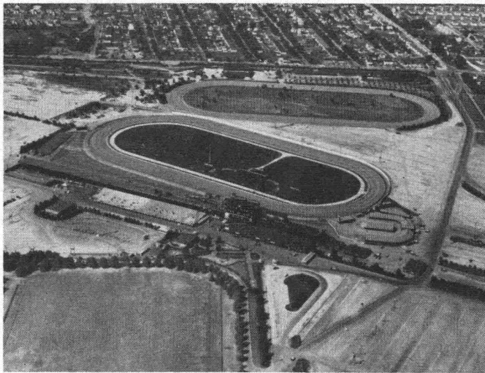
FIG. 4. Oblique view of racetrack installation which is being mapped photogrammetrically.
