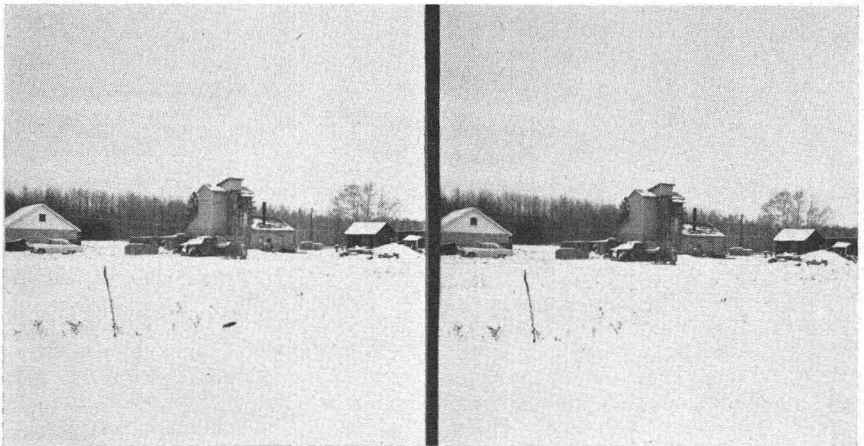
FIG. 4. The cement block plant. Washed sand and gravel are loaded into the tower and progress to the mixer and molds by gravity. Stacks of blocks appear on the other side of the plant. Aspen appears in the background. Dec. 1954. (Ed Steigerwaldt.)
