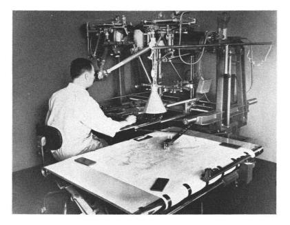
The diapositive is centered in the plate holding frame by a supplemental centering device which is furnished with the instrument. The plate holding frame can be moved closer to or farther from the projection center, and can be set at any distance from this center, between 125 mm. and 215 mm. This and other adjustments to the plate holding frame permits using cameras of focal lengths from 98 to 220 mm. Diapositives of any size up to  $9\frac{1}{2} \times 9\frac{1}{2}$ inches can be used.
