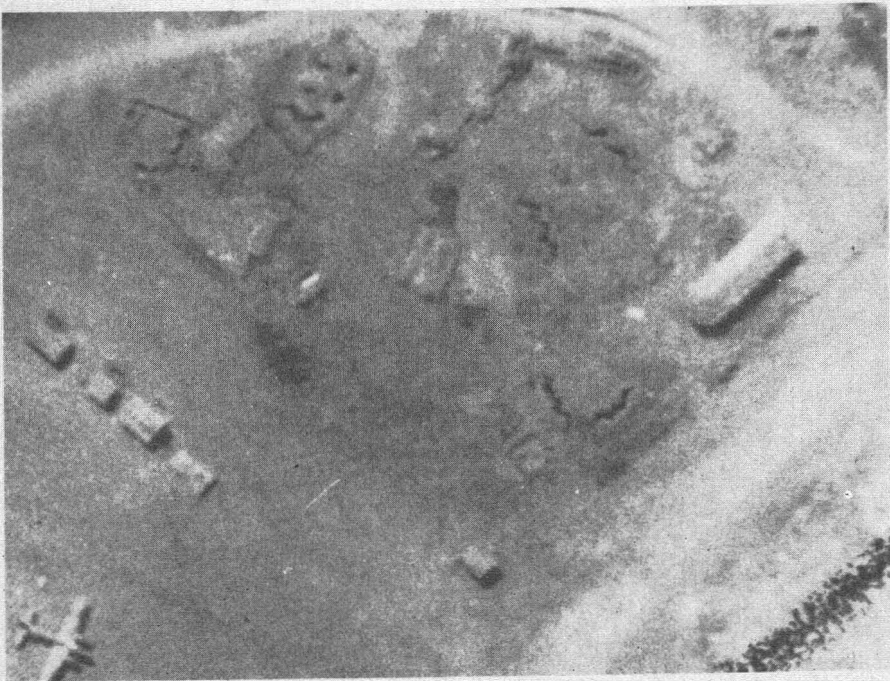
B. AERIAL PHOTO OF PERSONNEL TRENCHES AND OTHER AIRFIELD STRUCTURES
