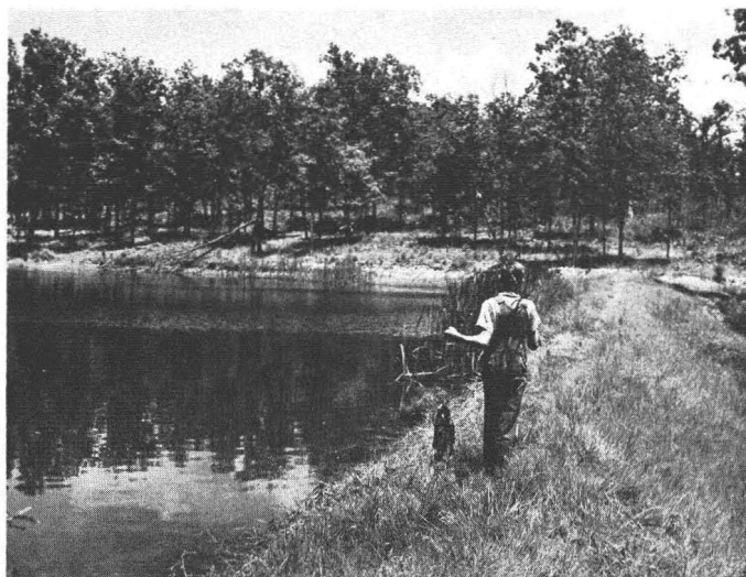
FIG. 3. This photograph shows part of a constructed pond of about the minimum size for recreational use. The boy in the picture is walking along the low earth dam, typical of those used to impound water for fishing, swimming, and boating, where natural water resources are not sufficient. (Courtesy of U. S. Soil Conservation Service).
