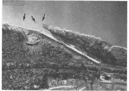
FIG. 8. Vertical Aerial Photograph, Heated Coolant Water Discharge Area, Dickerson (Maryland) Thermal Electric Plant.
