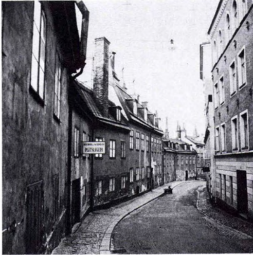
FIG. 3. A curved street including the fronts of 10 small buildings.
