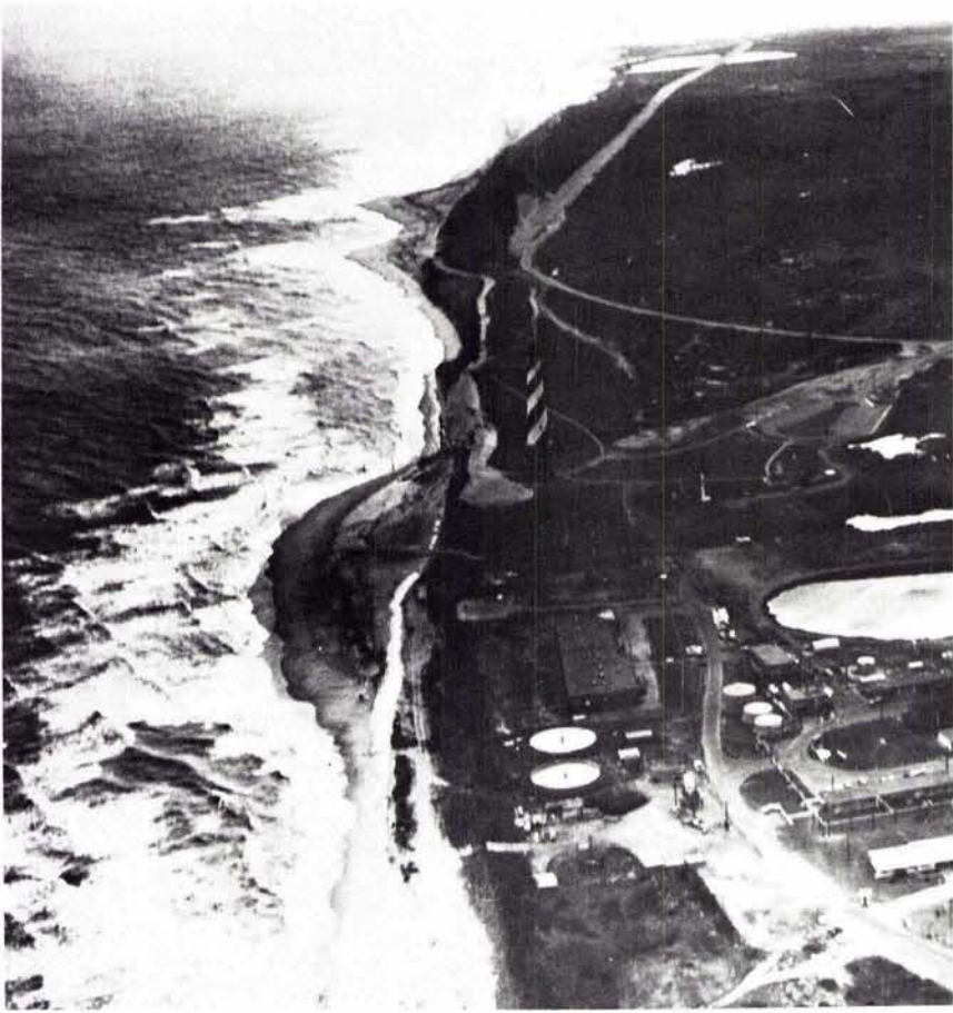
FIG. 2. Concern about erosion may depend upon the relation between the structure location and the sand wave position. The Cape Hatteras Lighthouse is vulnerable at the time of this photo, but the large mass of sand in the foreground will migrate toward the point and the Lighthouse will then be secure for a time.
