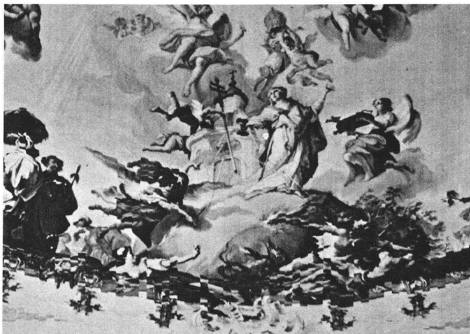
FIG. 2. Displacements at the border of a cupola caused by profiling errors.
