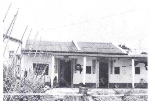
FIG. 5b. One-storied new village houses with double-sloping roofs and asbestos roofing.
