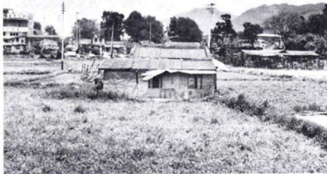
FIG. 4. Temporary shacks made of metal plates.
