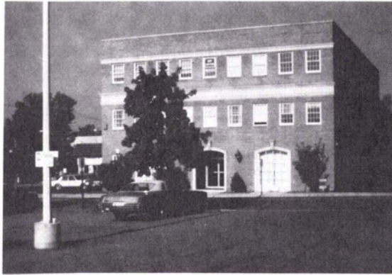
FIG. 4. ASP headquarters building.
