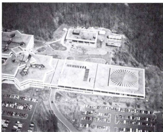
FIG. 3. Large resolution targets painted on the roof of the John Wesley Powell Federal Building, USGS National Center, Reston, Virginia.
