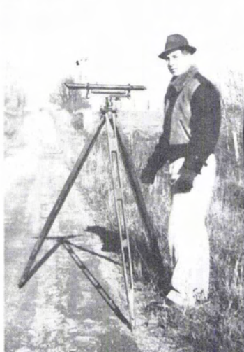
Joseph P. Burns working as an instrumentman on highway surveys in northern New York in 1938.
