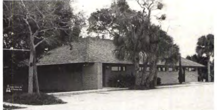
GSI facility in Melbourne, Florida designed by Duane Brown.
