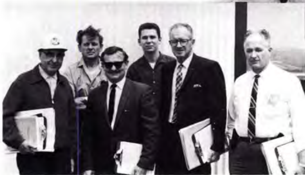
Inspection Team for sign-off of completed Tracking Radar Structures. USAF-RCA project. Half Moon Bay, Calif. Harry, at left, is Resident Engineer, 1967.
